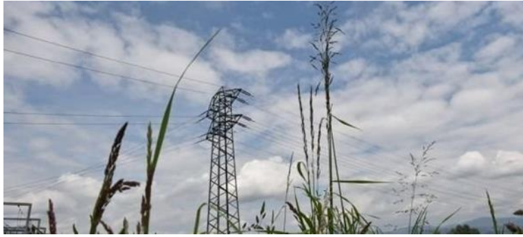
8 full size hydro electric power stations, 1578 gigawatt-hours consumption of traction current, 90% traction current from renewable sources
